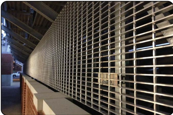
Aluminum Swaged Locked Grating used as security fencing
